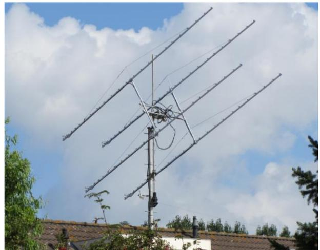
**PA2V's new 4 x LFA yagi array**
