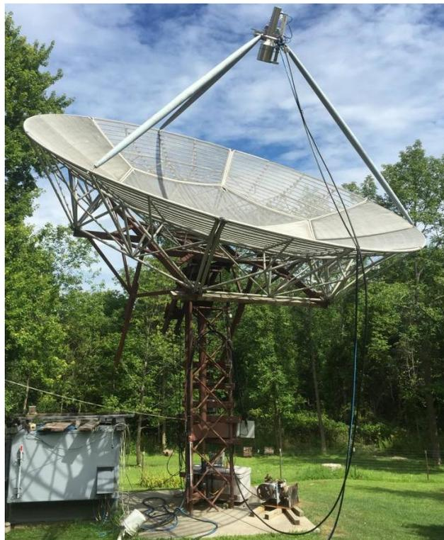
**WB2BYP's 28' dish with 23 and 9 (offset) cm feeds in place**
